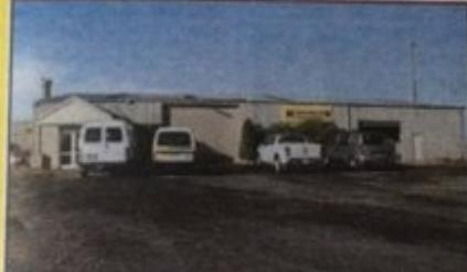
700m<sup>2</sup> shed plus 300m<sup>2</sup> lean to constructed of laminated timber Portal frame, timber rafters/purlins, 4.2m eave height, Colourbond steel roof & wall cladding in good condition.
