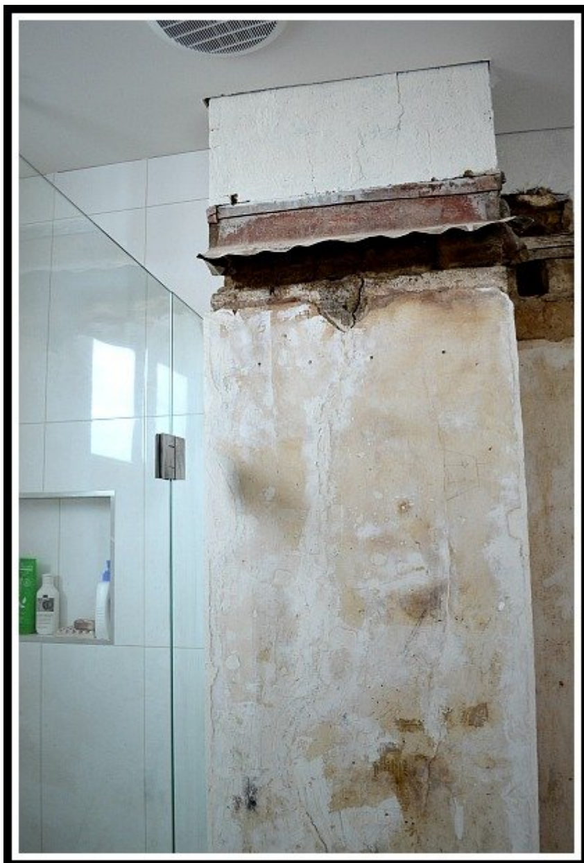
Old meets new: bits of original corrugated iron and rendered sandstone remain a feature of the very modern ensuite.
