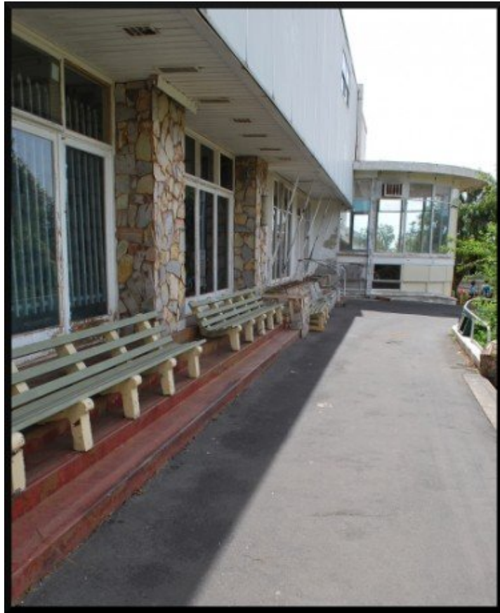
Building details, Fletcher Jones factory complex, Warrnambool.
