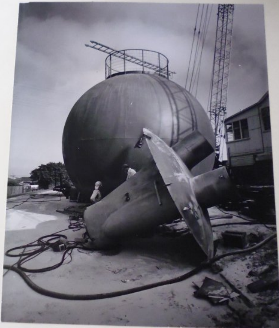
THE SPHERICAL TANK IMMEDIATELY BEFORE ERECTION. THE BOTTOM CROWN PLATE IS IN THE FOREGROUND, COMPLETE WITH PART OF THE INNER TANK AND ATTACHED EXTENSIONS OF THE TOWER COLUMNS.
