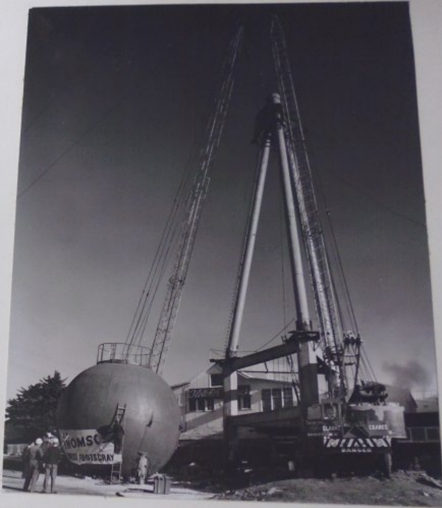
BOTTOM CROWN PLATE ASSEMBLY IN PROCESS OF BEING FASTENED TO THE TOWER COLUMNS.
