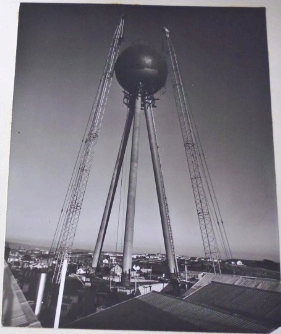
FINAL POSITIONING OF THE SPHERICAL TANK DURING THE ERECTION PROCESS.
