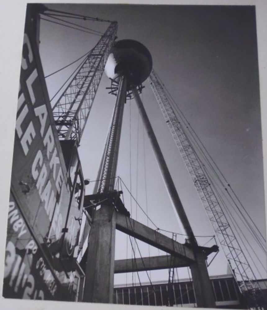
SPHERICAL TANK IN PROCESS OF BEING LIFTED ON TO THE BOTTOM CROWN PLATE ASSEMBLY.
