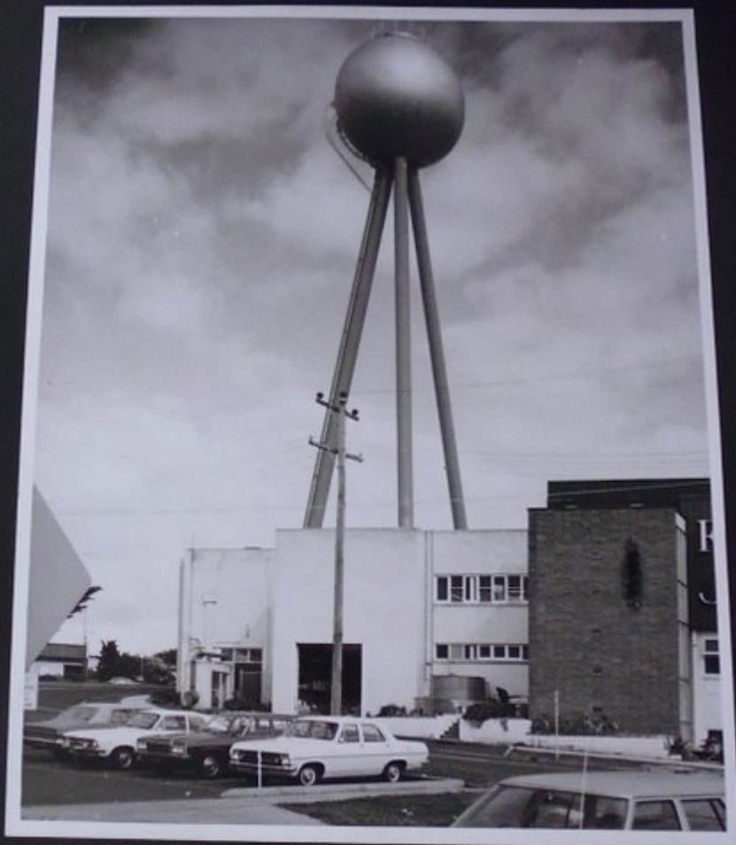
THE COMPLETED TWO-STORY FACTORY EXTENSIONS INCORPORATED WITH THE WATER TOWER BASE.
