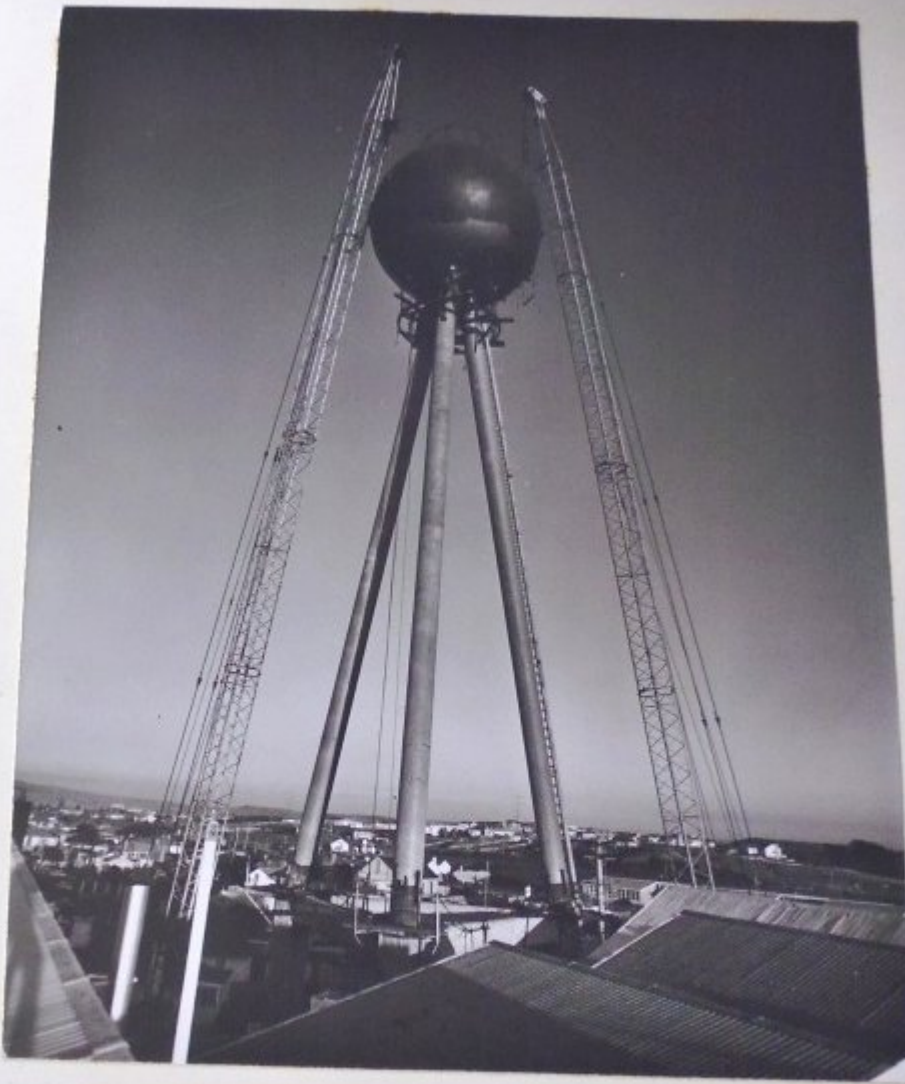
FINAL POSITIONING OF THE SPHERICAL TANK DURING THE ERECTION PROCESS.
