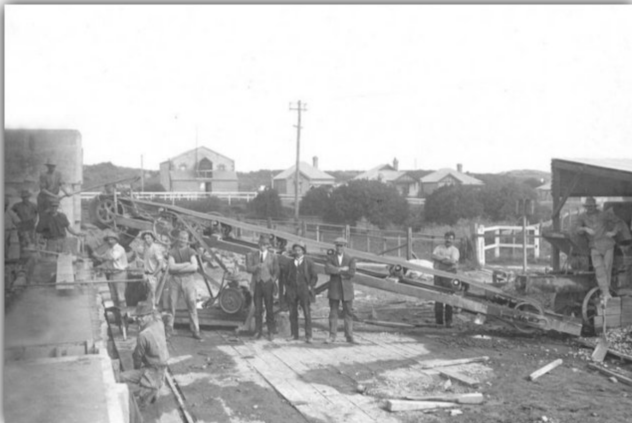
The Stanley St bridge can be seen in the backdrop of this photo taken in 1890, showing workers at a railway reserve unloading huge concrete blocks that would be used to build the breakwater. Image: Warrnambool Historical Society.
